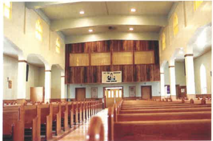
View from altar, Oct 1987, just prior to reconstruction
