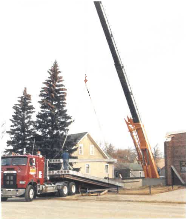
Dec. 1/87 Crane at work - still no snow
