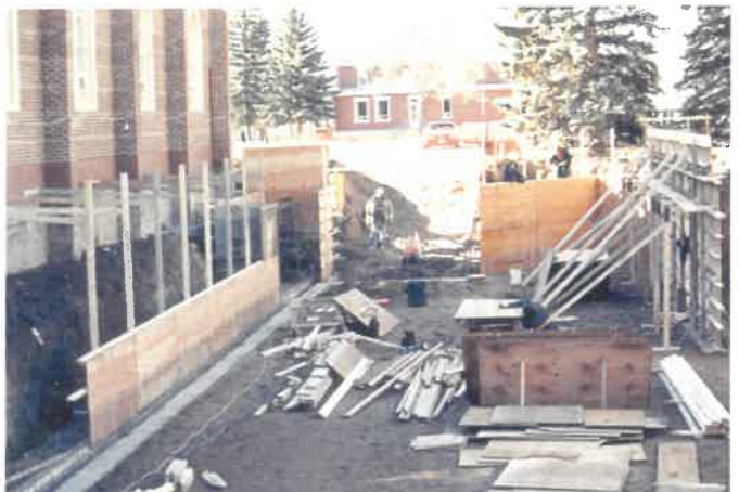
Nov 24/87 Basement walls go up
