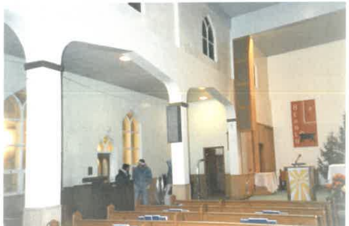
Front left, Oct 1987, prior to reconstruction
