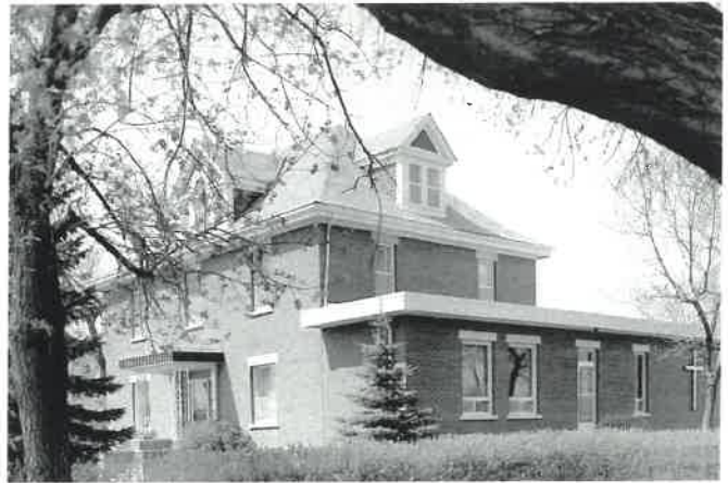
Sisters of Loretto Convent, view from SE. Photo from Loretto Archives, Loretto Abbey, Toronto
